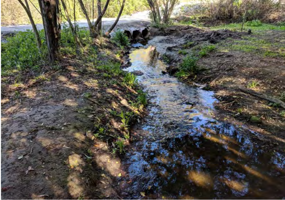
13 - OHWM 2A-1, low-flow channel facing northwest (downstream)
