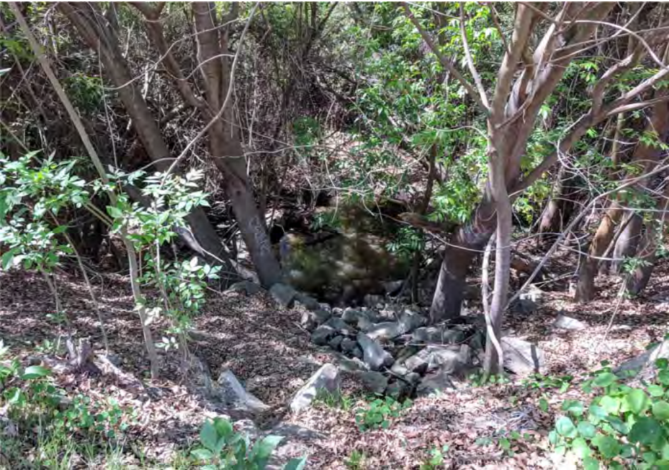
23 - Outfall area facing southwest
